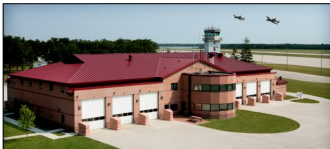
Above: Alpena CRTC Fire Station and Control Tower with two A-10s overhead. (photo courtesy of: alpenacrtc.ang.af.mil )
